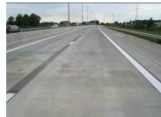
The design strives both for durability and sustainability, with Continuously Reinforced Concrete Pavement being noted for its long lifetime combined with concern for the environment and the finite nature of natural resources. This project may therefore be most certainly regarded as an optimised sustainable road design.
